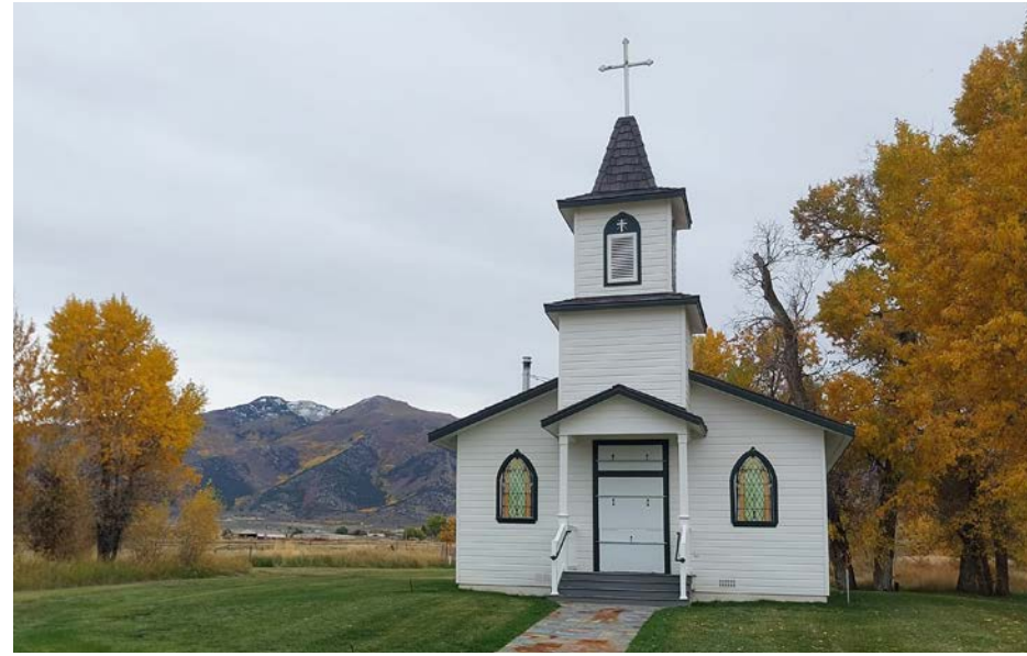
Photos courtesy of Foundation 36
